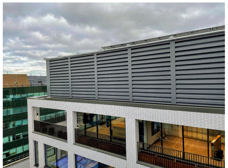
Figure 4 - Acoustic Louvre Screen.
